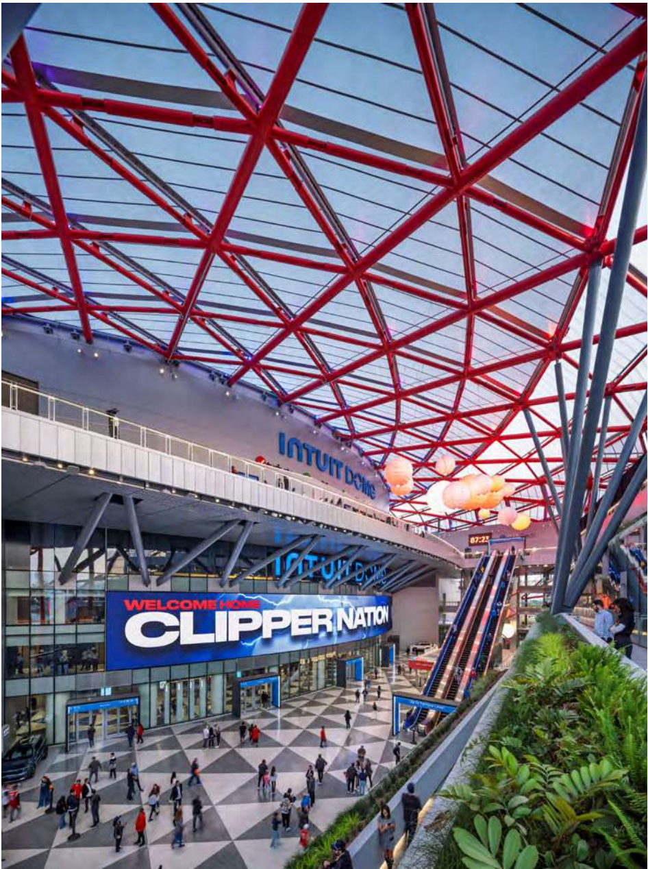
Intuit Dome. Photo credit: Tim Griffith
