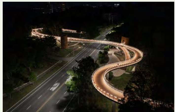
Zhuhai Banzhang Mountain Footbridge
