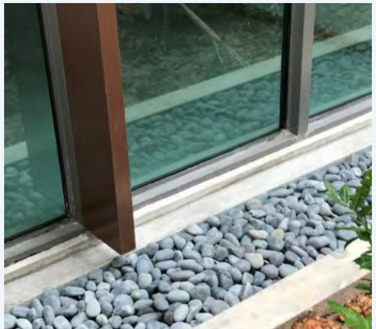
Figure 4: Positioning soil/planted areas away from glazed surfaces reduces its frequency of cleaning
