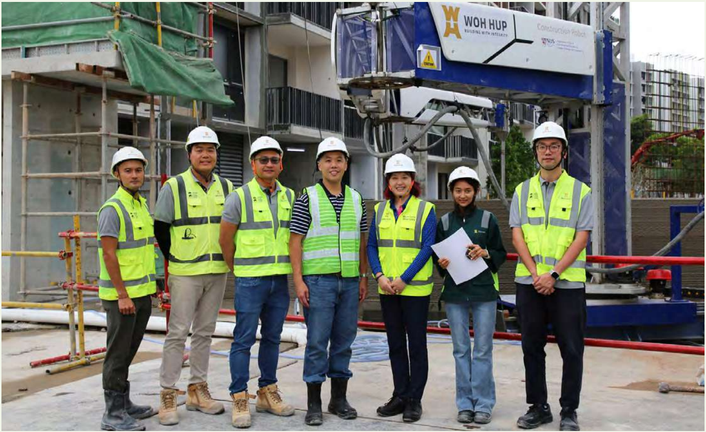
NUS Associate Professor Pang Sze Dai (4th from left) with Er Cong Zhengxia (5th from left) and collaborators from Woh Hup at an on-site 3D concrete printing exercise, validating the newly developed approach under real-world conditions. Photo credit: College of Design and Engineering at NUS
