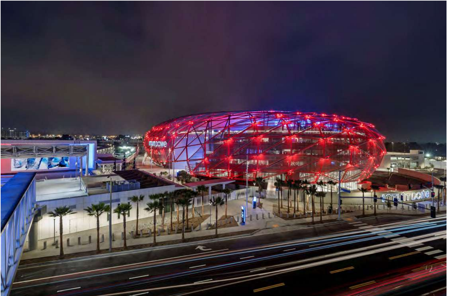
Intuit Dome. Photo credit: Tim Griffith
