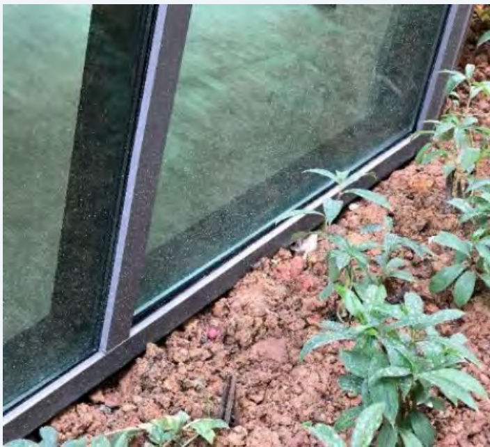
Figure 4: Positioning soil/planted areas away from glazed surfaces reduces its frequency of cleaning
